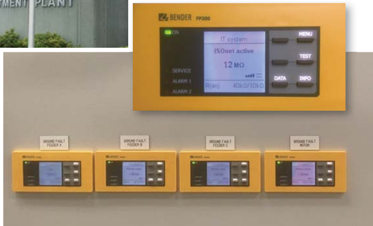
FP200 display and operator unit for devices of the iso685 series without display
