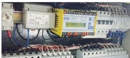
Due to these considerable advantages – maximum safety at minimal cost – the installation of the collection storage is implemented with two unearthed IT systems. Both the AV system (normal power supply) and the SV system (safety power supply), were built as three-phase AC systems and are monitored by means of an ISOMETER<sup>®</sup> from the series IRDH260. In the SV system the control of the fire alarm system and CO<sub>2</sub> extinguishing system are continuously monitored.
