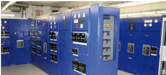
Electrical installation at NürnbergMesse
