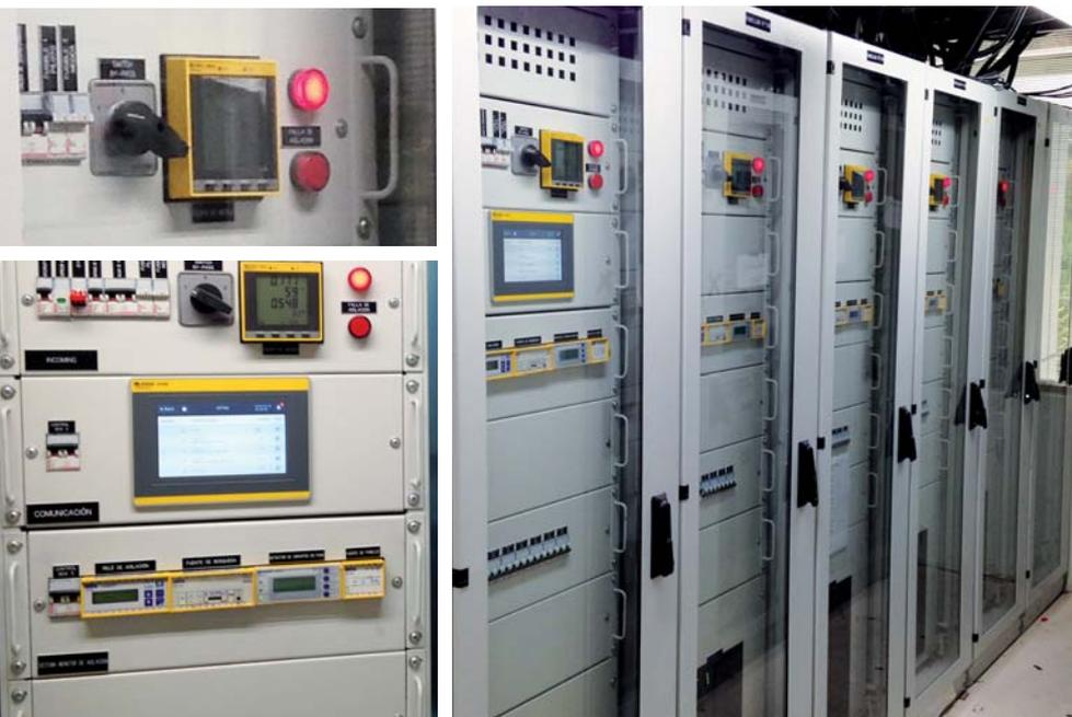
lation fault location in group two rooms by Bender, residual current monitoring for TN-Systems by Bender, power quality analysers by Bender and Condition Monitor CP700. All devices are integrated in the CP700 touch control panel for convenient system handling and overview.
