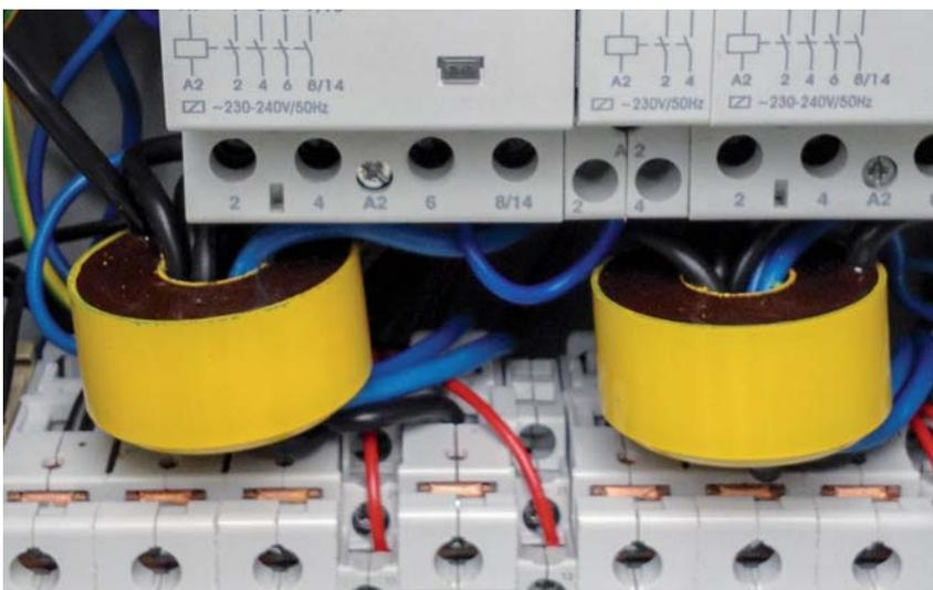
Figure 6: RCMB 420 EC 2 channels
