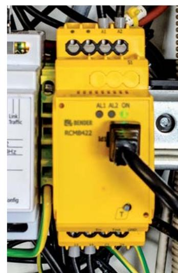
Figure 7: RCMB 420 EC 1 channel
